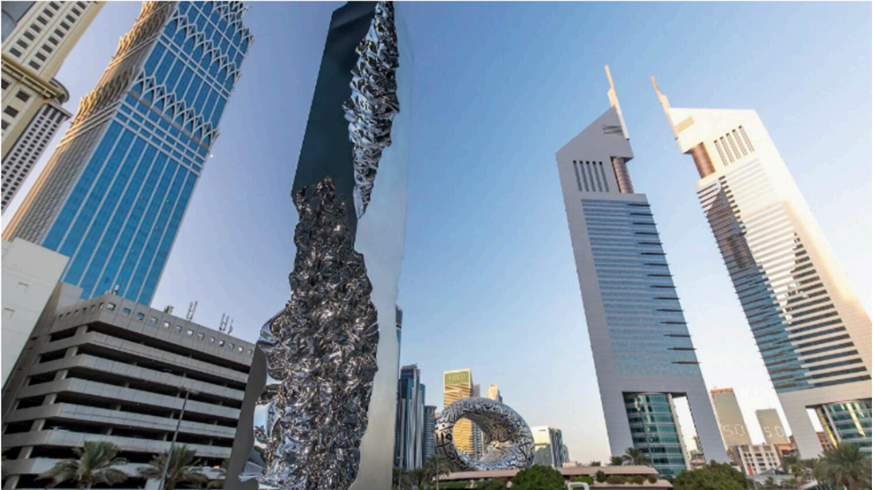
Pillar of Fortitude at DIFC
